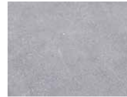
Coloured Concrete with Broom Finish.
