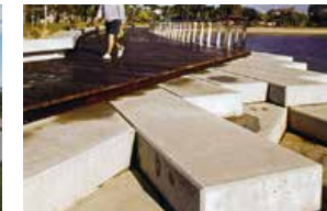
Access to Water: Formed concrete
