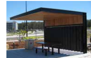
Shelters: Powder-coated steel framing and hardwood timber
