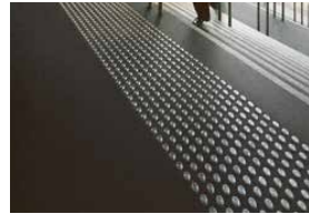
Tactile indicators: Stainless steel with grit insert ground surface indicator dots
