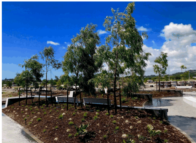
Stage 1A1 - urban square works
