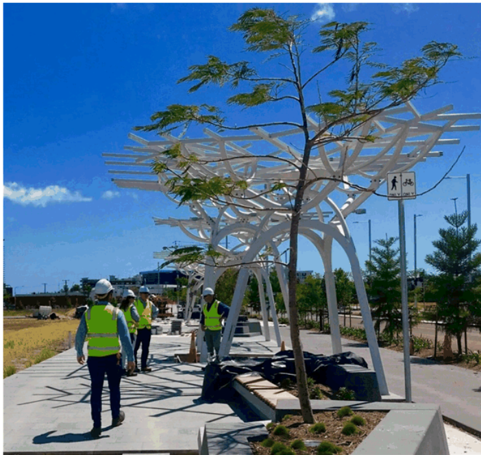
Stage 1A1 – First Avenue works
