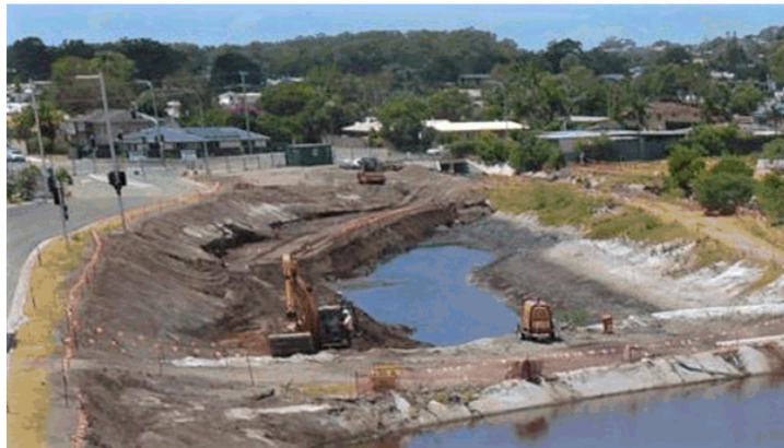
Stage 1A2 - East Corso works
