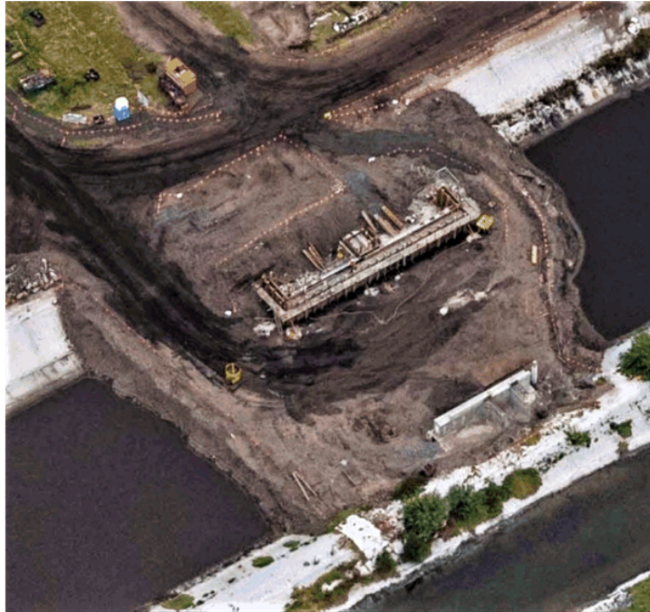
Stage 1A1 - bridge abutment works Mundoo Blvd Bridge (across Corso)
