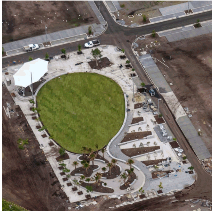
Stage 1A1 - urban square works
