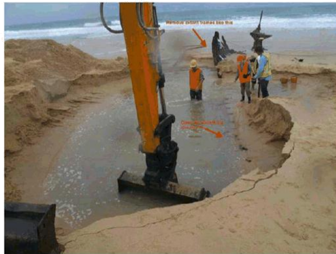
Figure 43. Example of where frames are to be cut down to on starboard side. The stubs in the foreground are the tips of the floors, the frames having been removed by recent storm surges. (Cosmos Archaeology, 28 April, 2014)
