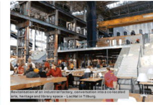
Revitalisation of an industrial factory, conversion into a co-located arts, heritage and library space - Localt in Tiburg.
