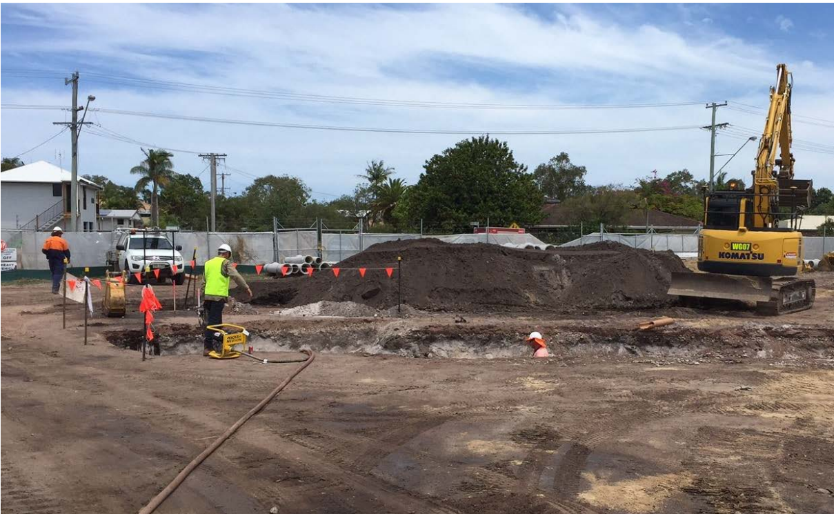
Image 2: Commencement of Maud Street intersection works
