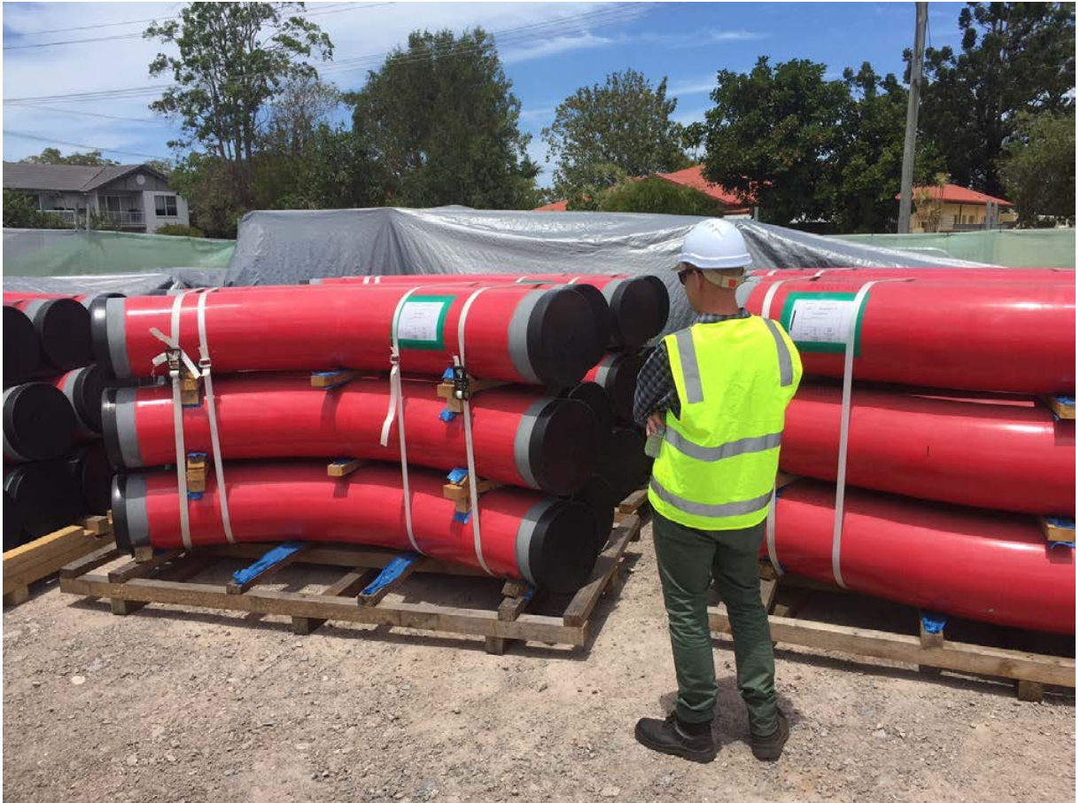
Figure 4: Shipment of AWCS pipes delivered to site
