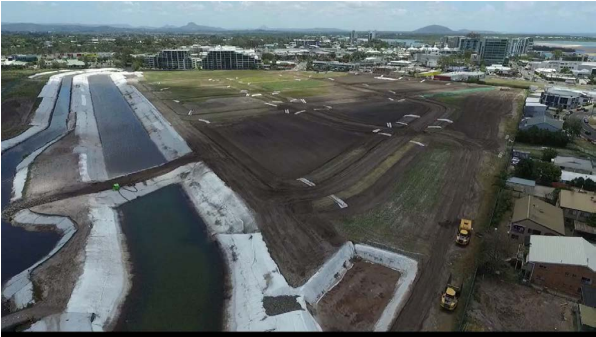
Image 1: Completion of Stage 1A bulk earthworks, November 2016
