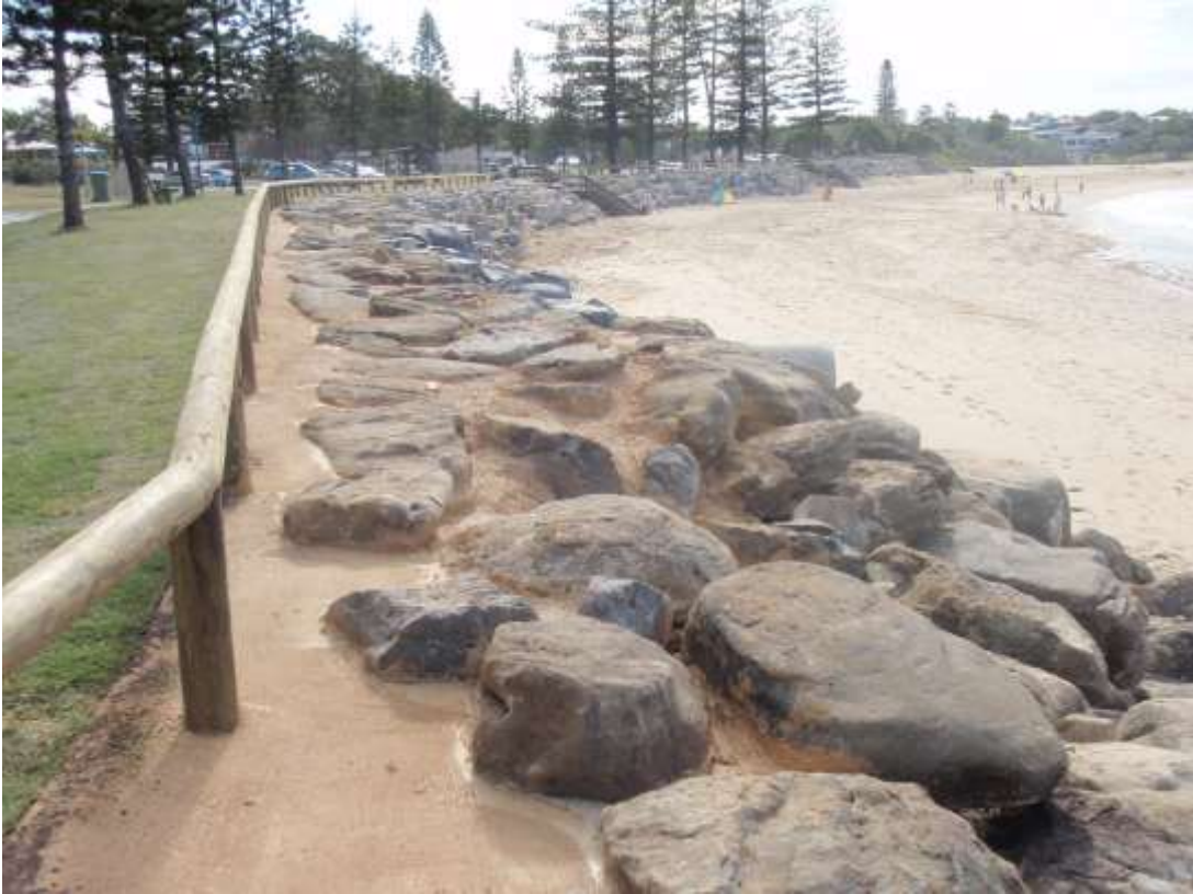
Photo 2 Completed seawall Moffat Beach (Oct 2008)
