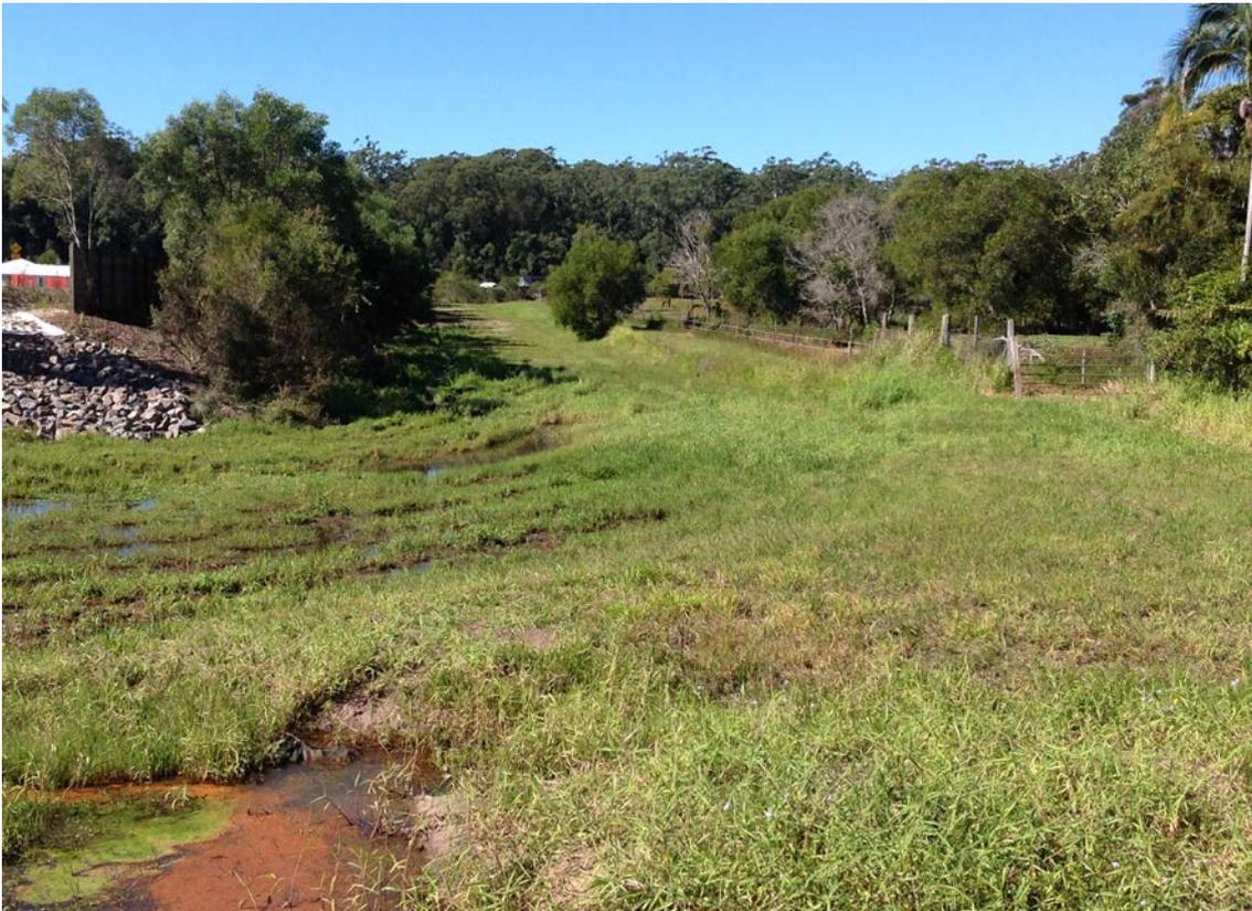
Figure 12 Poor Open Channel –Ponding, odour, weed incursion, unable to be maintained (source: Switchback Consulting)
