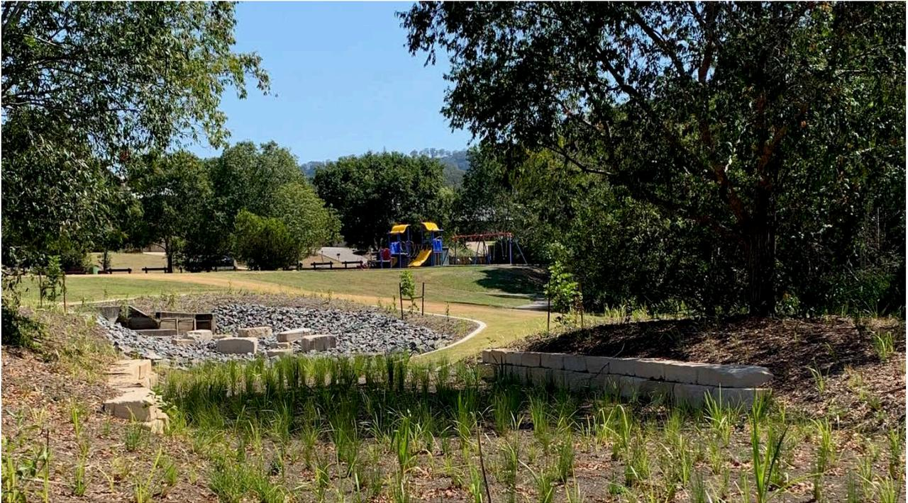
Figure 3 Complementary co-location of bioretention basin (source: Sunshine Coast Council)
