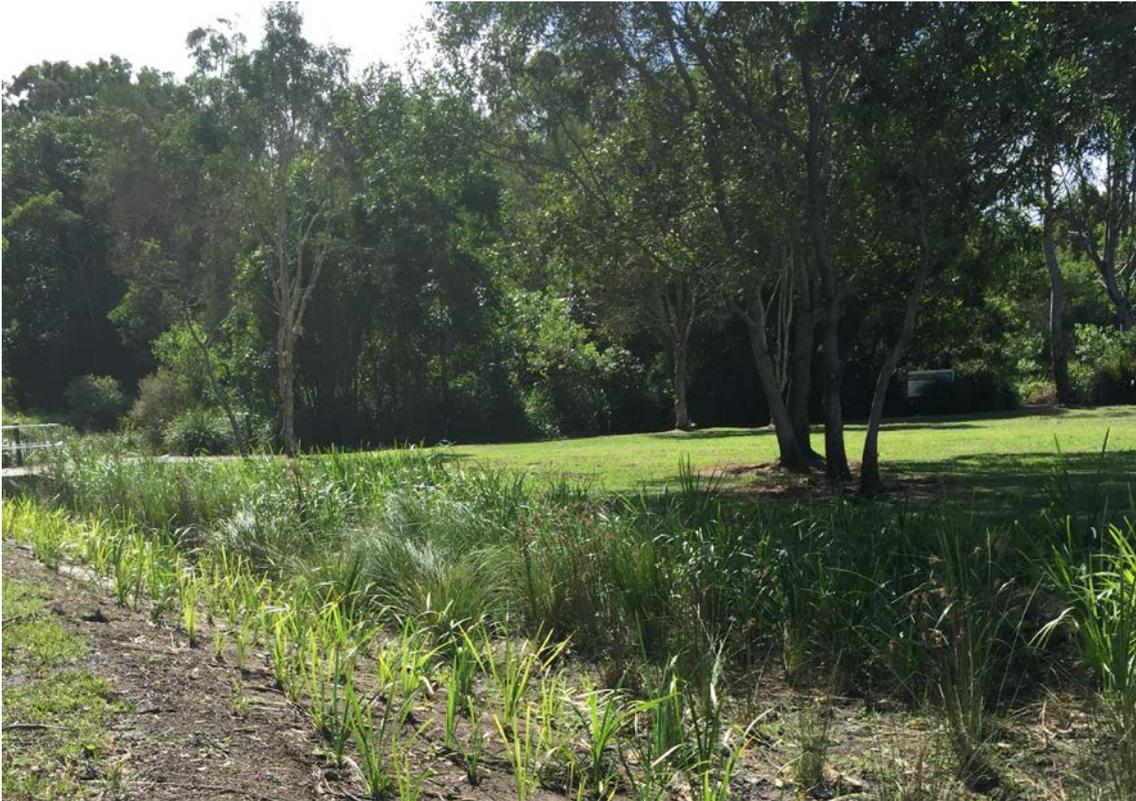
Figure 13 Better Open Channel –Free draining, densely planted, coir mat stabilisation during establishment, shading (source: Switchback Consulting)
