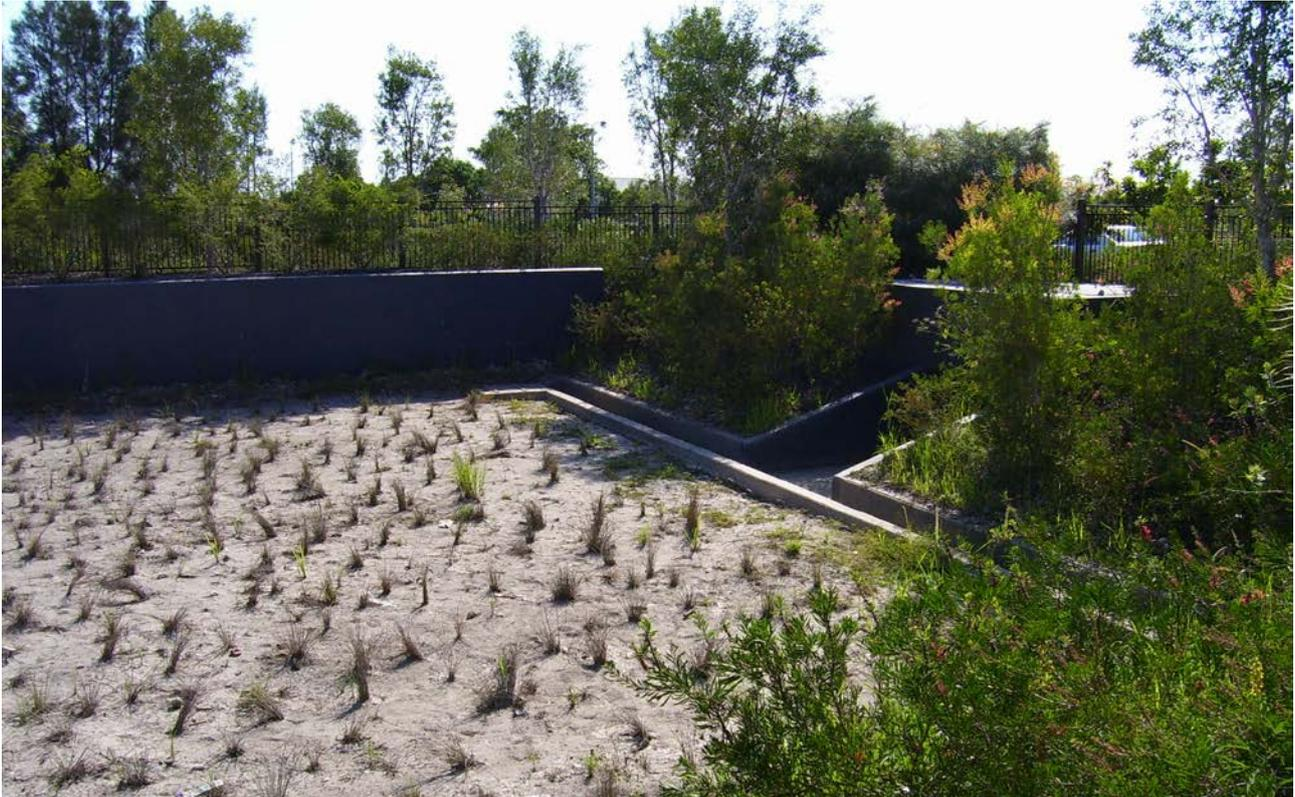
Figure 2 Poorly integrated bioretention basin (source: Switchback 48 Consulting)
