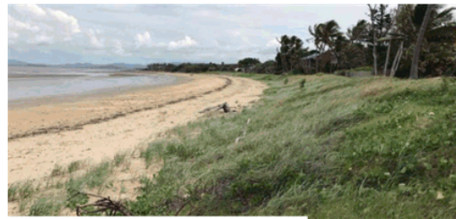
Buried geo-bag seawall at Zilzie, QLD
