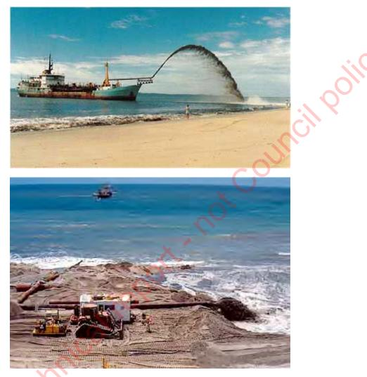
Figure 2-7 Rainbowing at Woorim Beach (top panel, BMT WBM, 2014) and Pumping Sand Onshore (bottom panel, SANDAG, 2015)
