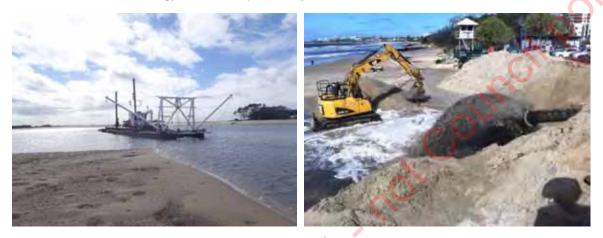
Figure 2-20 Cutter Suction Dredge and Pipeline Sand Delivery to Maroochydore Beach
