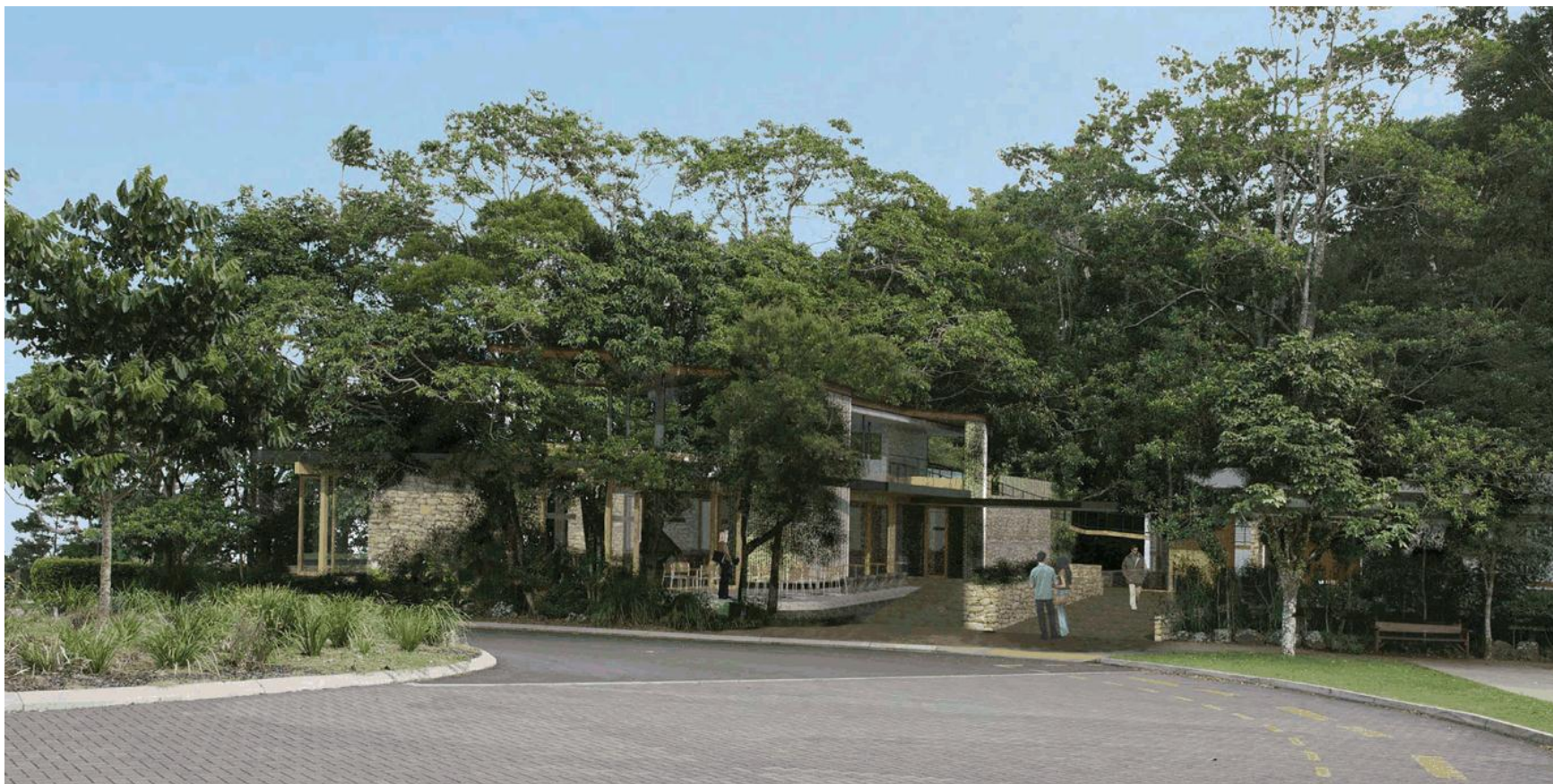
VIEW 1B - FROM EXISTING CAR PARK
