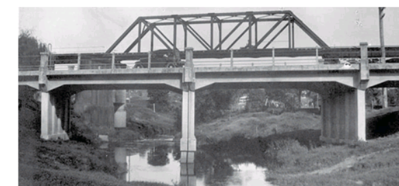
Currie Street bridge cir 1935
