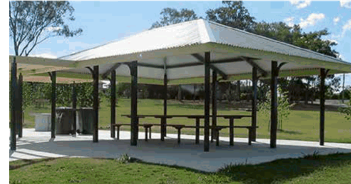
Hip style shelter roof
