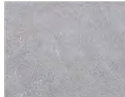
Coloured Concrete with Broom Finish.
