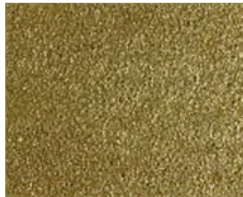
Integrally Coloured Concrete with Lightly Exposed Aggregate
