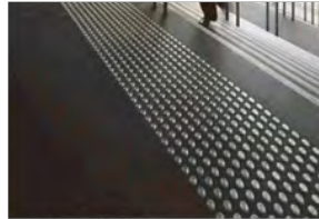
Tactile indicators: Stainless steel with grit insert ground surface indicator dots
