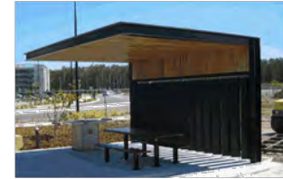
Shelters: Powdercoated steel framing and hardwood timber
