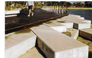
Access to Water: Formed concrete
