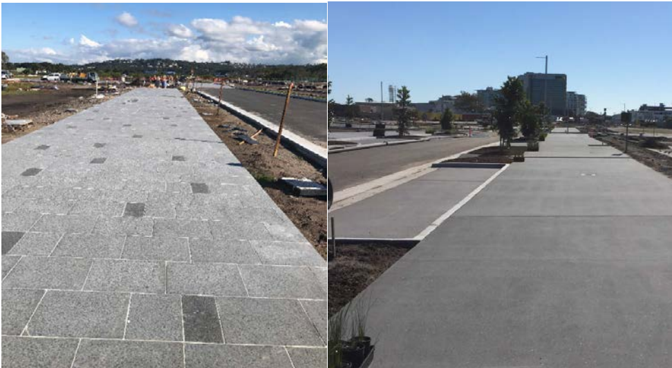
Stage 1A footpath paving and street plantings
