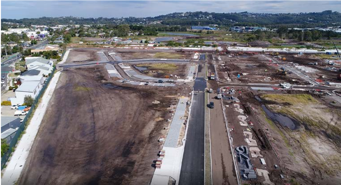
Stage IA Works
