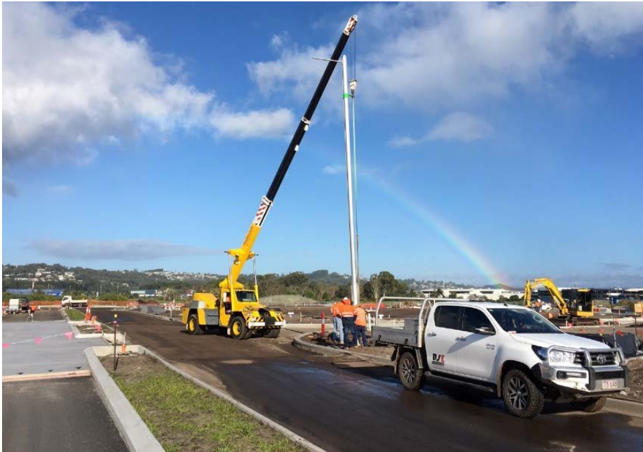
Stage 1A installation of street lighting
