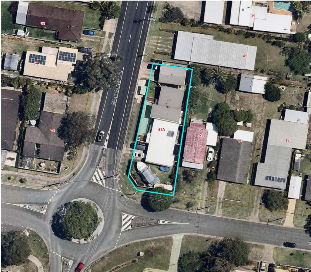
Figure 3: Aerial image of site
