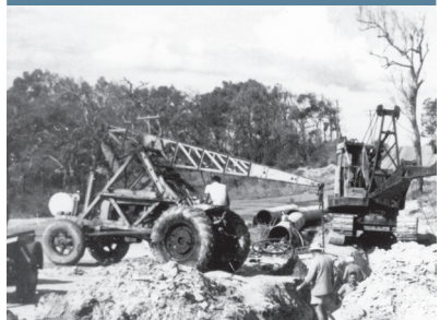
Caloundra water tower and pipes being installed at Queen Street, ca 1965
