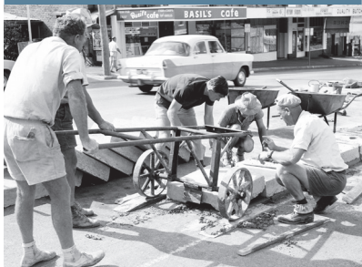
Road workers installing a traffic island in Currie Street, Nambour, 1966
