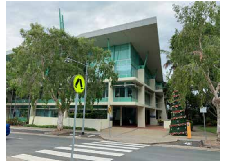
Caloundra Administration Building 2019
