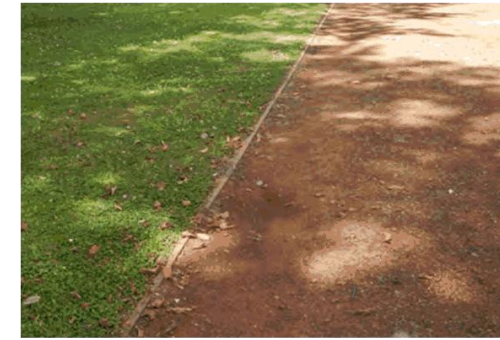
Timber Edging - Buggy Shed / Paths / new Gardens - Treated or seasoned / recycled HWD timber Refer Schedule on L03
