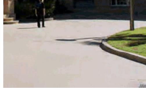
Rear Path from House Concrete slab – fine broom finish, – colour: standard grey, or red oxide Alternative: a plain, non-textured concrete paver
