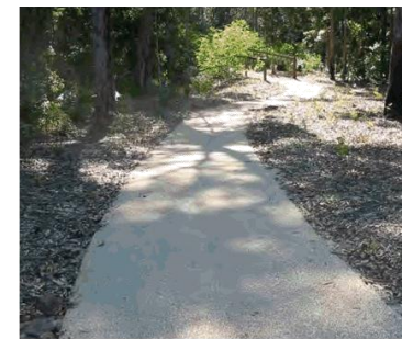
Front Path Restoration, Main Paths & Buggy Shed Area - Option: - 'Bushmates' bituminous gravel - colour: Autumn Gold supplier: Bushmates
