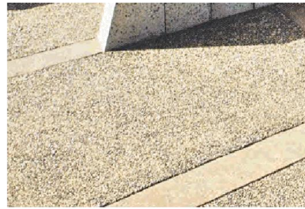
Rear Path from House Concrete slab – fine broom finish, – colour: standard grey, or red oxide Alternative: a plain, non-textured concrete paver
