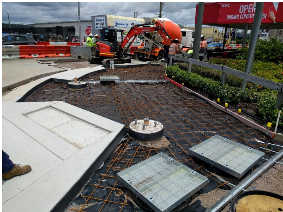
Aerodrome Rd North West Road Verge Construction
