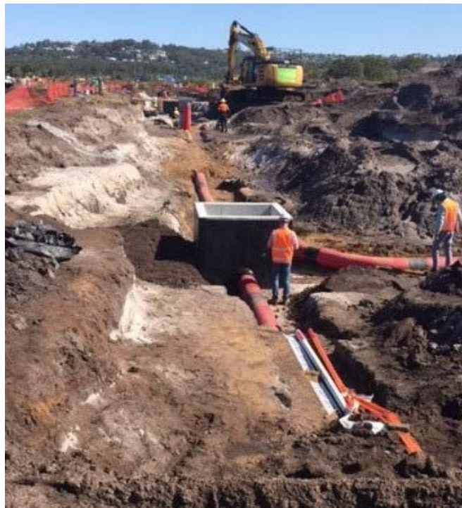
Stage 1A – AWCS installation
