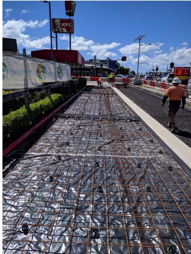
Aerodrome Rd North West Road Verge Construction
