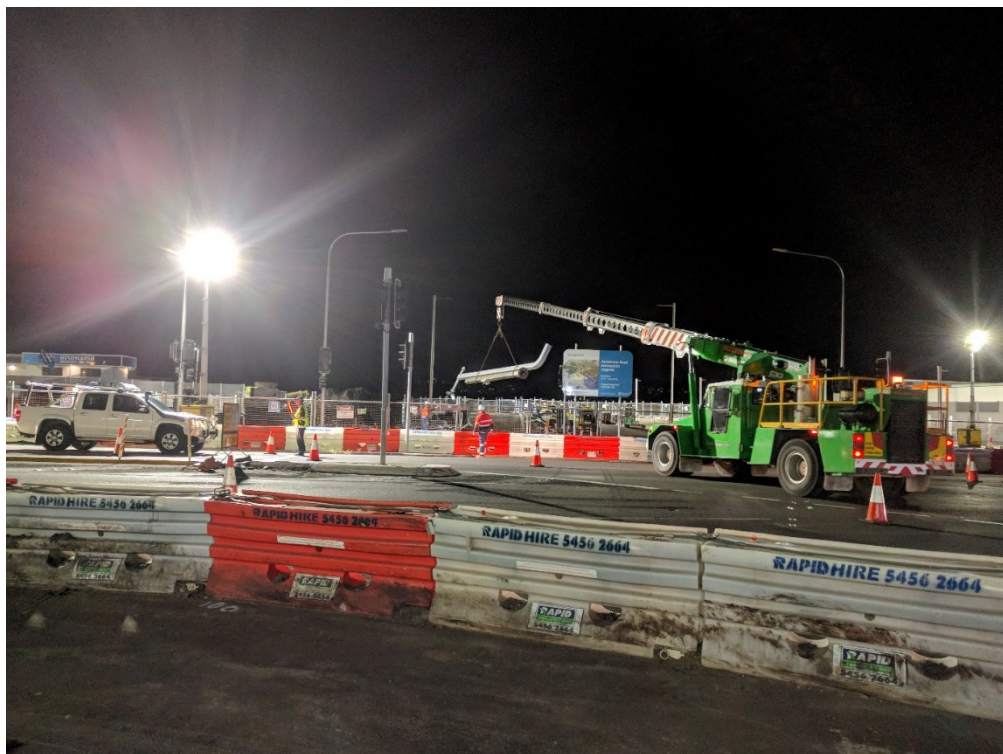
Installation of Traffic Signals and Light Poles during Nightworks
