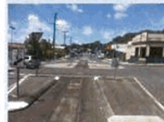
Tracks pass through the William Street roundabout on Howard Street.
