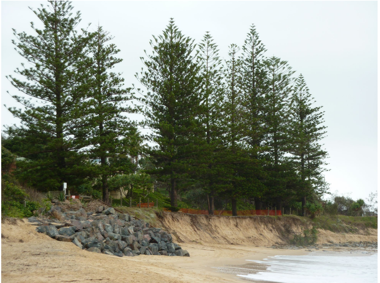
Figure 1: Previous erosion, existing seawall and Norfolk Pines – Cooroora St dunal system
