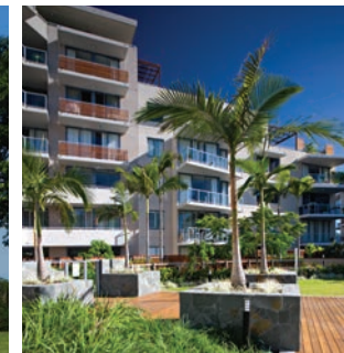
Medium rise tower and podium 8 - 15 storeys (200-250 dwellings / Ha) 30 - 45m height limit sites
