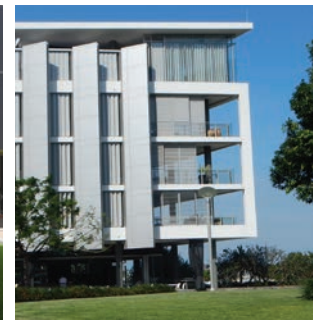
Low - medium rise, lift apartments 4 - 8 Storey (120-150 dwellings / Ha) 15 - 25m height limit sites
