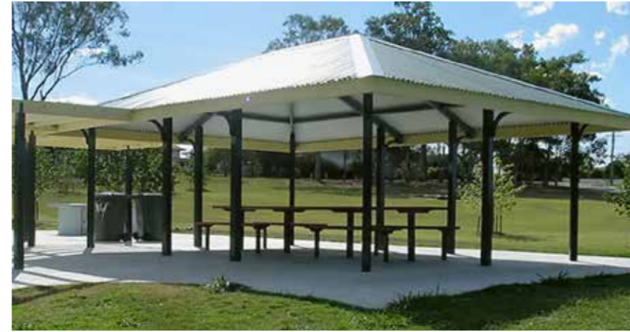
Hip style shelter roof
