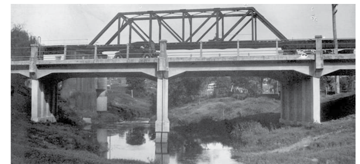
Currie Street bridge cir 1935
