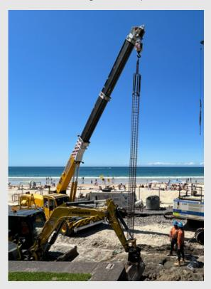
**Piling finished:** Once all piles are in place, the guide wall is removed. The excess concrete material is reused as fill behind the seawall.
