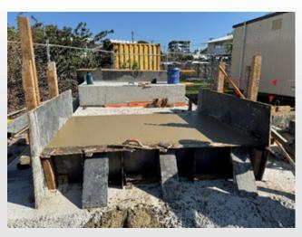
**Formwork:** Each terraced step uses steel formwork moulds to create the shape of each terrace. These steel moulds are then reused throughout the seawall terrace construction. *Image above right, shows the steel formwork being removed after the concrete has cured.*
