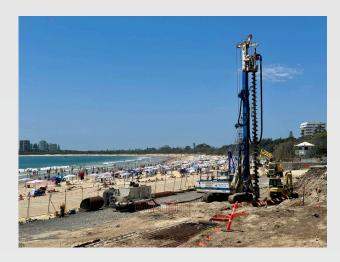
**Primary piles installed:** As the drill comes up, concrete is pumped into the hole created by the drill to form the first set of piles. These piles extend up to 5 metres below ground level and form the start of the wall below ground.
