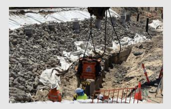
**Building the seawall terraces:** Plain concrete is poured to create a 'blinder' which provides a working platform to allow for the concrete terraces to be constructed. Steel moulds (formwork) are then used to create the exposed fronts of the terraces and seating areas.
