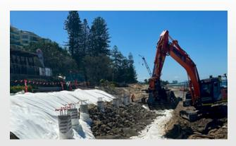
**Preparation for lowest terrace:** The tops of the piles are then cut back to expose the reinforcing using a device called a 'cropper'. Steel reinforcement is then prepared to connect with the first level of the seawall terraces. See below image of the 'cropper' in action.
