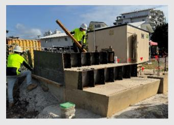
**Example seawall:** Construction starts from the lowest level terrace (which will be buried under sand) and moves upward towards the parkland and Esplanade level. *Image below shows an example of the seawall's terraced steps and shows the plain concrete 'working platform' beneath the sand coloured terraces.*
