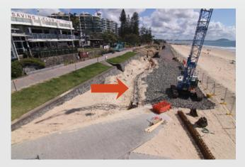
**Bringing in the piling rig:** Specialist construction machinery is required to install the piles. The drill has a spiral blade that rotates and buries into the ground. As it drills down, it pulls up and removes the soil/sand. *Image below of the piling rig in action*.
