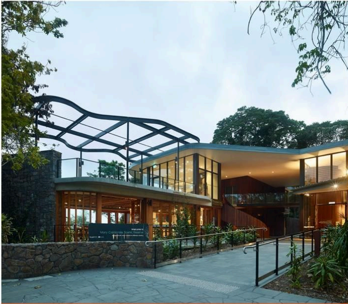
P 01 The building layout is in two parts linked by a breezeway that captures natural breezes. The building opens to the north to capture natural light and to the south to capture views.
