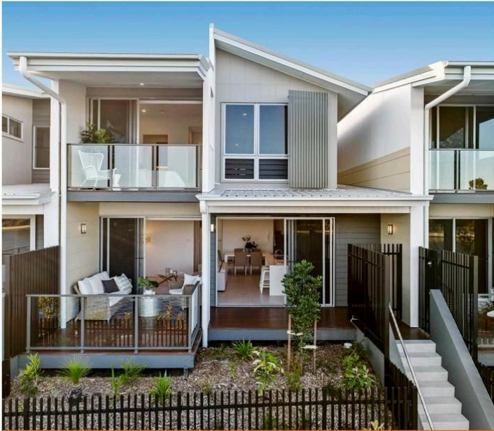
P 01 The design utilises climate control systems that are easy for residents to use, including operable windows, sun shading and screens and ventilated light wells that create a heat stack effect, where air gets warmer and typically rises naturally, ventilating the building.
