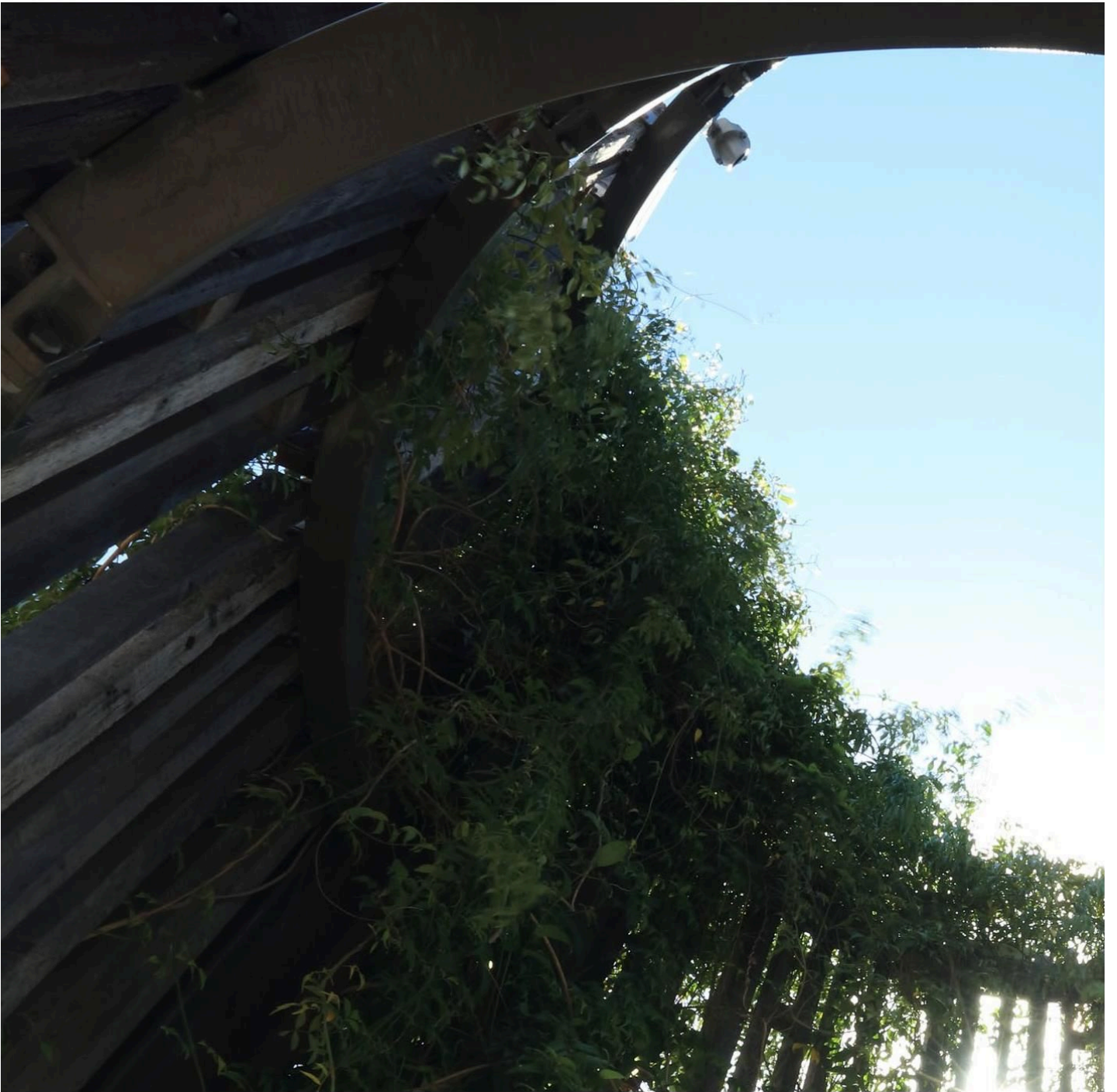
Understanding the local history and people through community engagement inspired the distinctive tower design.
