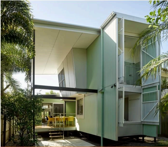
P 01 The inclusion of large windows and doors allow walls to open up and capture local breezes.
