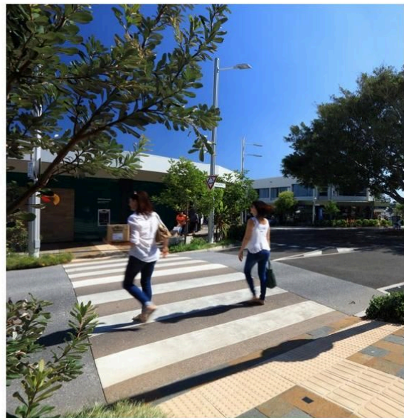
P 08 Flush kerbs provide a continuous accessible street surface for all pedestrians. Natural stone paving provides visual and textural wayfinding at crossings and intersections.
