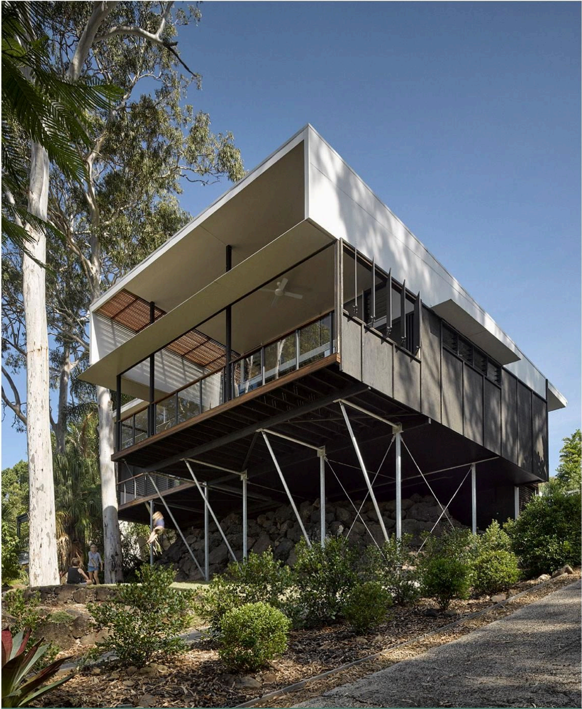
P 09 The design employs a lightweight steel structure, which ensures the development 'touches the ground lightly', respecting and minimising impact on the established landscape. This lightweight construction lends itself to future modification and adaptation, creating a place that is resilient and ready for change.
