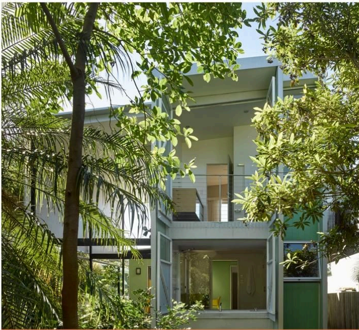
P 02 The renovation and extension retains existing trees and planting on site.
