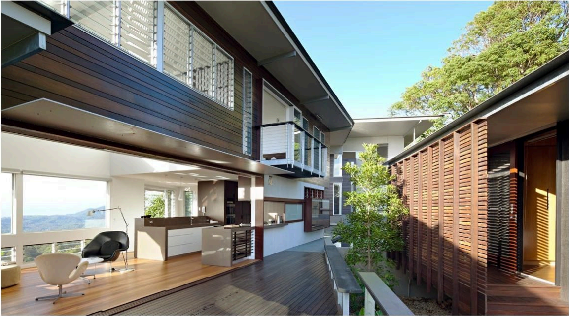
Doors, windows and screens are aligned to allow breezes to flow through the house, reducing the need for air-conditioning.
