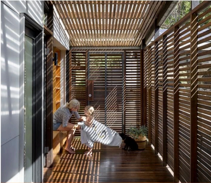
P 01 The central 'breezeway' corridor and veranda support easy movement between the indoors and outdoors and allow good cross ventilation through the building. They allow natural light into the internal spaces and offer sun-shading where required.
