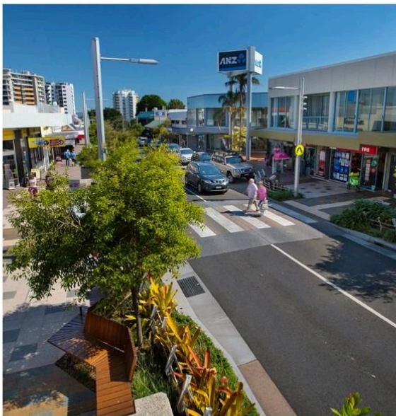
P 07 Telecommunication, gas, power and water services are accommodated underground to 'free up' the street for pedestrians, shade trees, street furniture and cafe seating.
