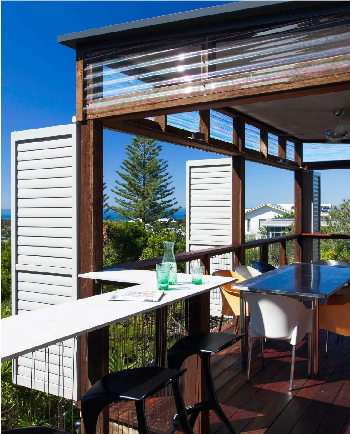
Doors, windows and screens can be opened and closed to harness and control natural breezes and provide protection from unfavourable weather all year round.
