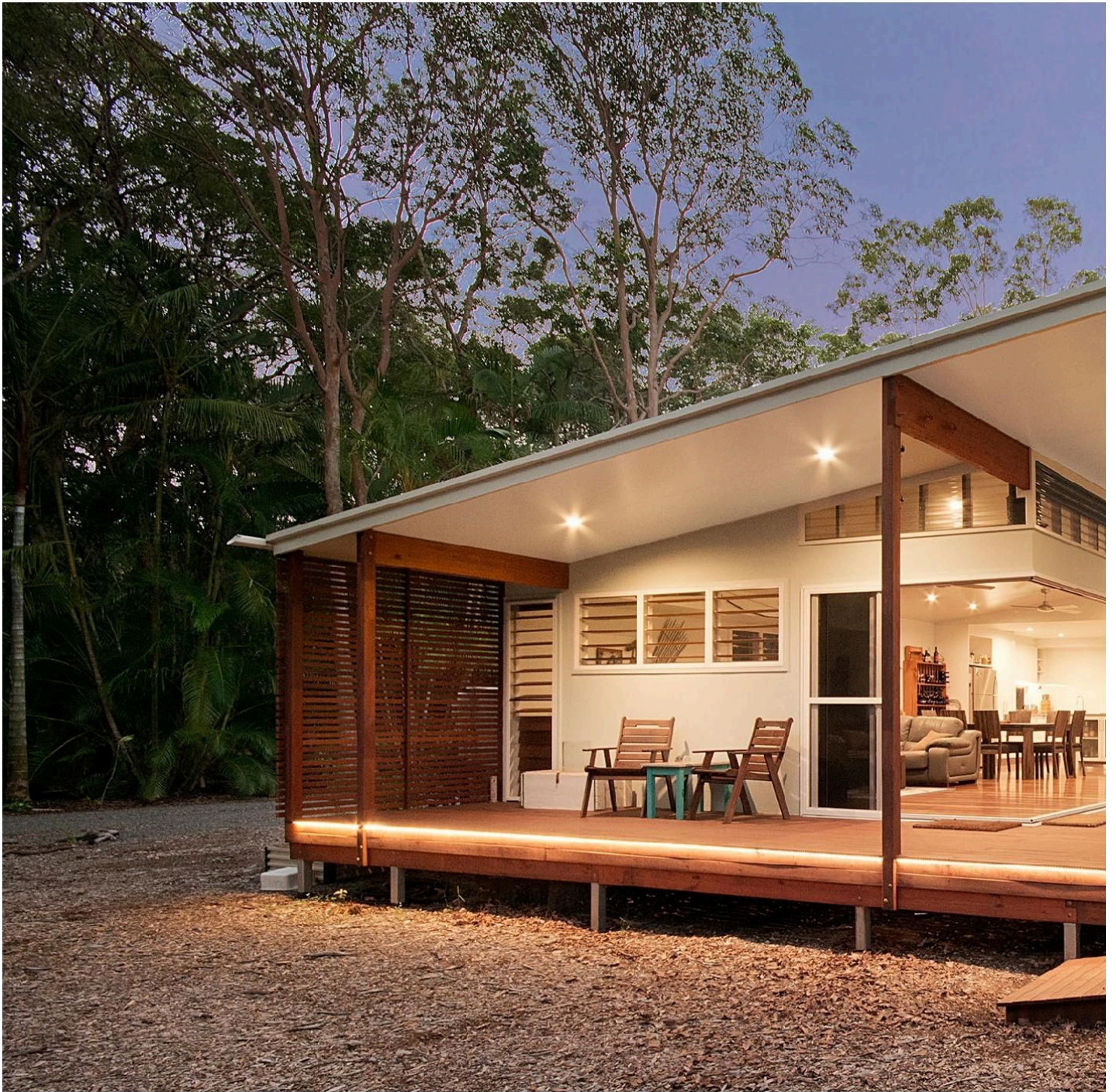
Doors and windows are located to provide visual and physical connections between indoor and outdoor spaces, making the most of the subtropical climate.
