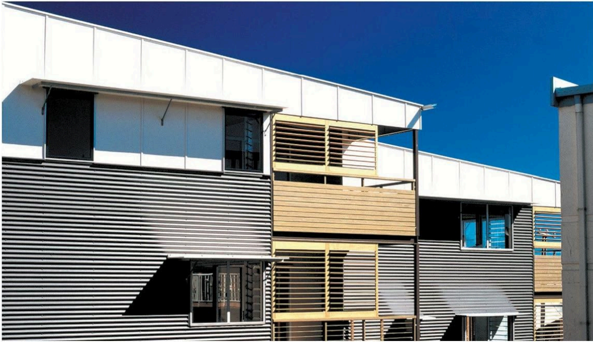
Battens covering fibro sheet cladding joints are a contemporary reference to pre and post war housing construction.
