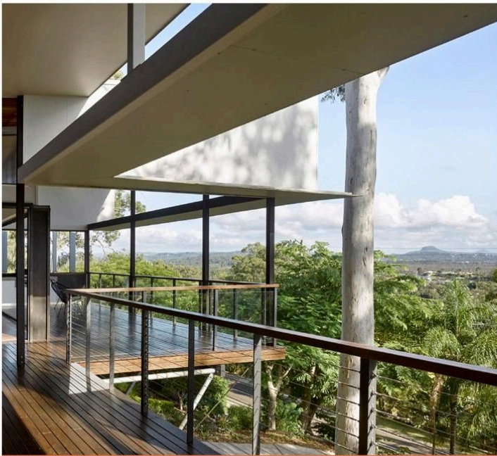
P 02 The house design preserves the location of two existing flooded gum trees by building around them, and adopts them as a focal point and connection to the natural landscape setting.
