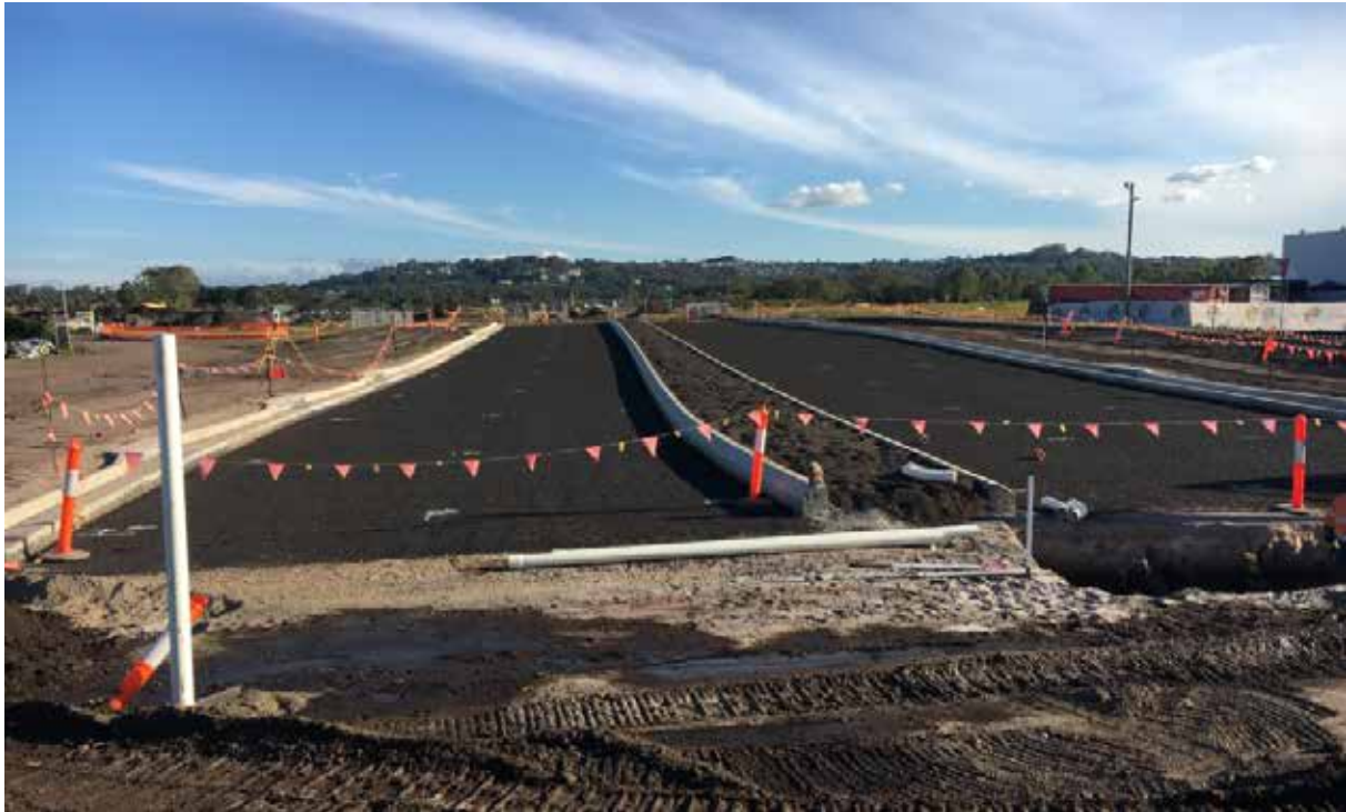
Partly complete Town Centre Boulevard (TCB) – Looking South
