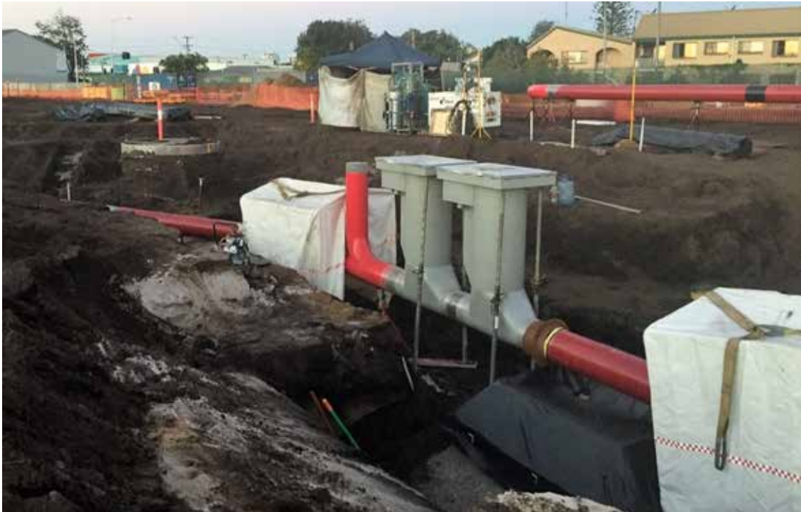
Figure 1. AWCS pipework being installed as part of Stage 1A
