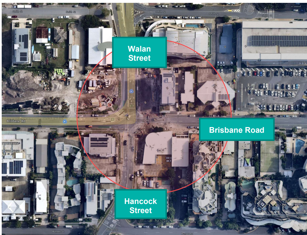
Figure 1. Night works construction areas* – 4 – 11 August 2022
