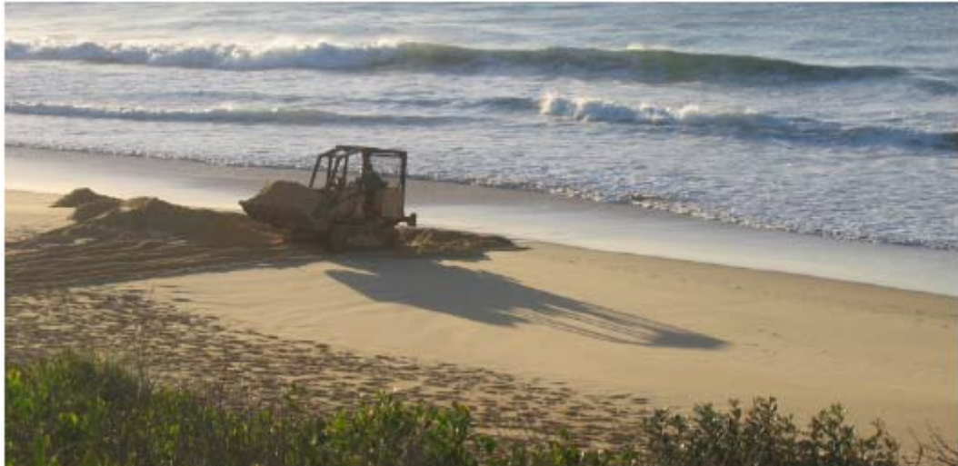
Figure 3-1 Beach Re-profiling using Mechanical Equipment (Source: Carley et al., 2010)
