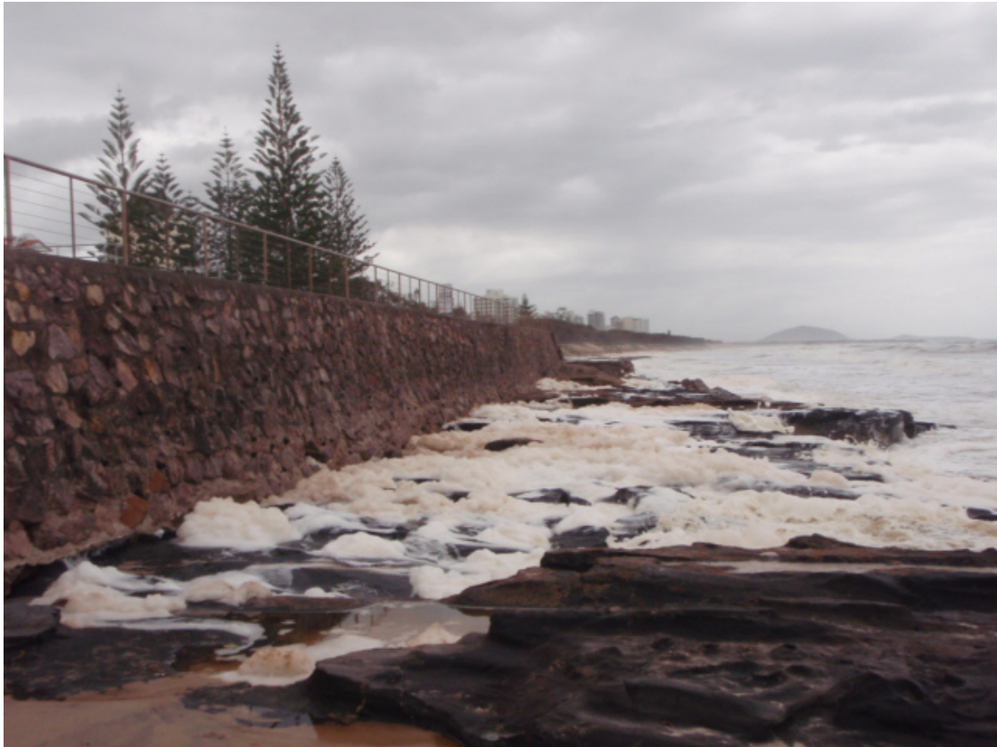
Figure 3-4 Seawalls on Eroding Shorelines Cause Loss of Usable Beach
