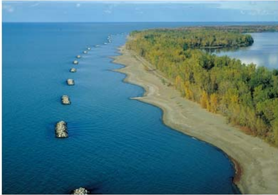
Figure 3-6 Offshore Breakwater Series and Salient Formation (Source: U.S. Army Corps of Engineers, 2002)
