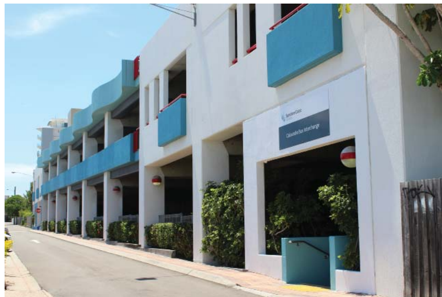
Caloundra Bus Station
