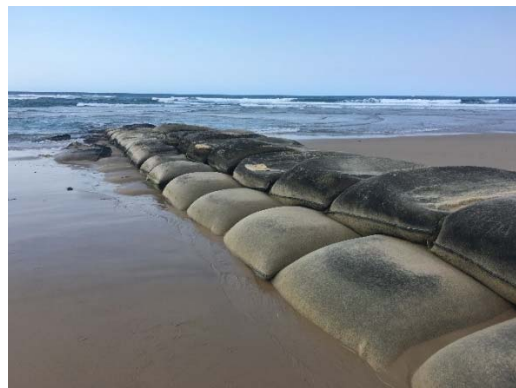
Figure 3: GSC style groyne (SCC, 2017)
