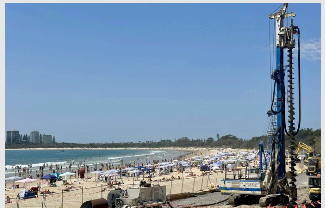
Stage 2 construction and seawall foundation piling rig.
