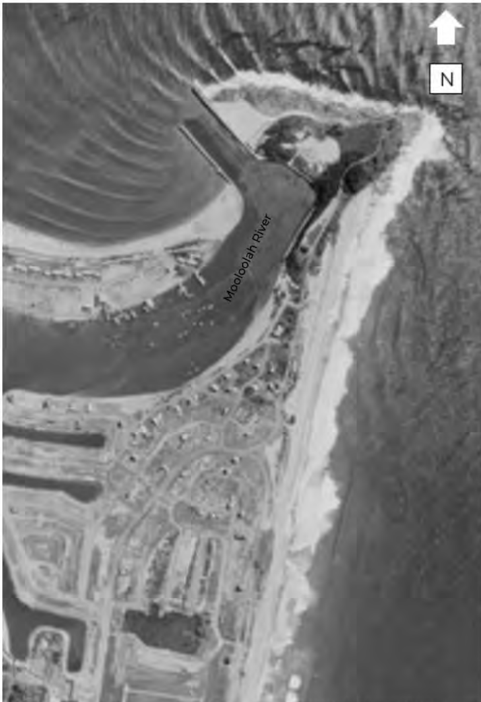
Figure 8: Aerial photo from May 27 th , 1971, QAP2230009 (QImagery 2022).
