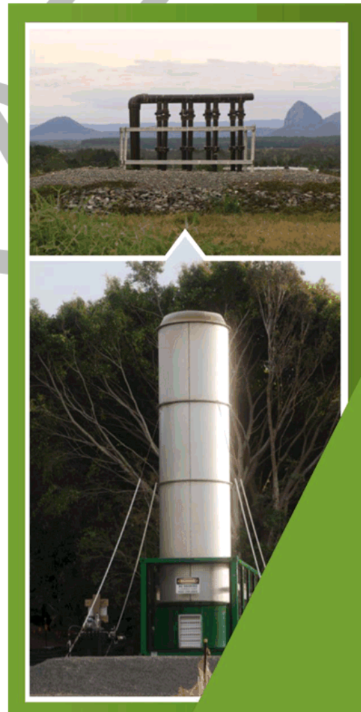
Images (Top to bottom, left to right): Image 16: Caloundra landfill gas manifold, Image 17: Caloundra landfill gas flare
