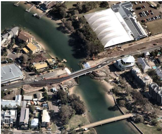
New Mayes Canal Bridge construction in progress
