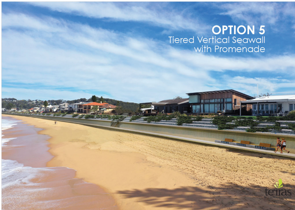
Figure 6.3 Terraced seawall option (not Mooloolaba, Terras, 2021)
