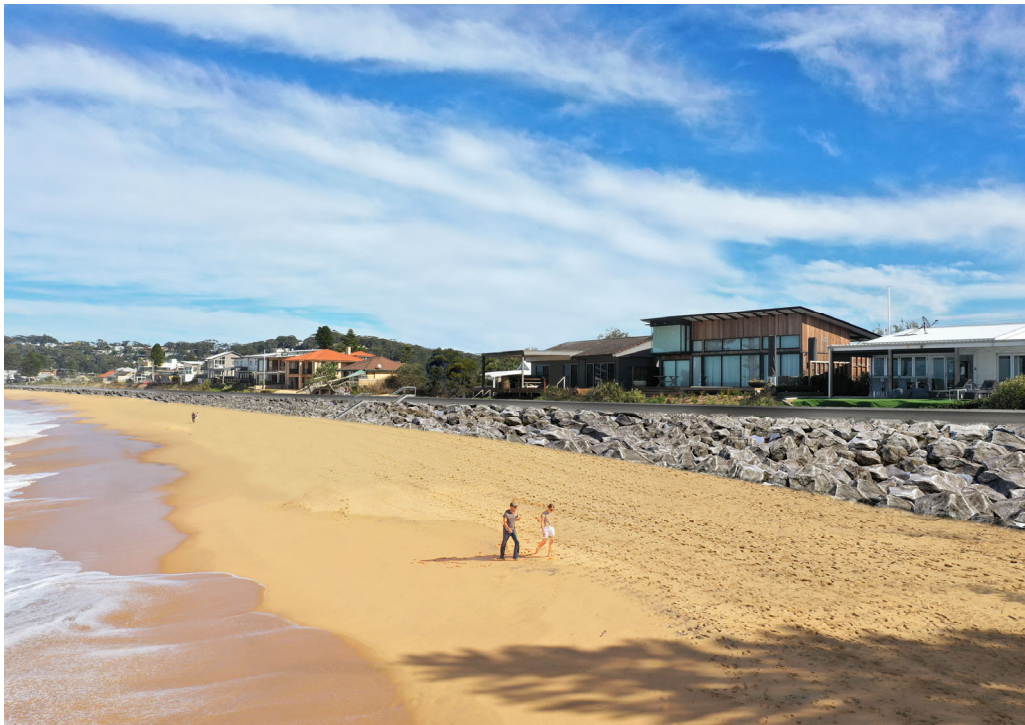
Figure 6.1 Rock rubble seawall option (not Mooloolaba, Terras, 2021)
