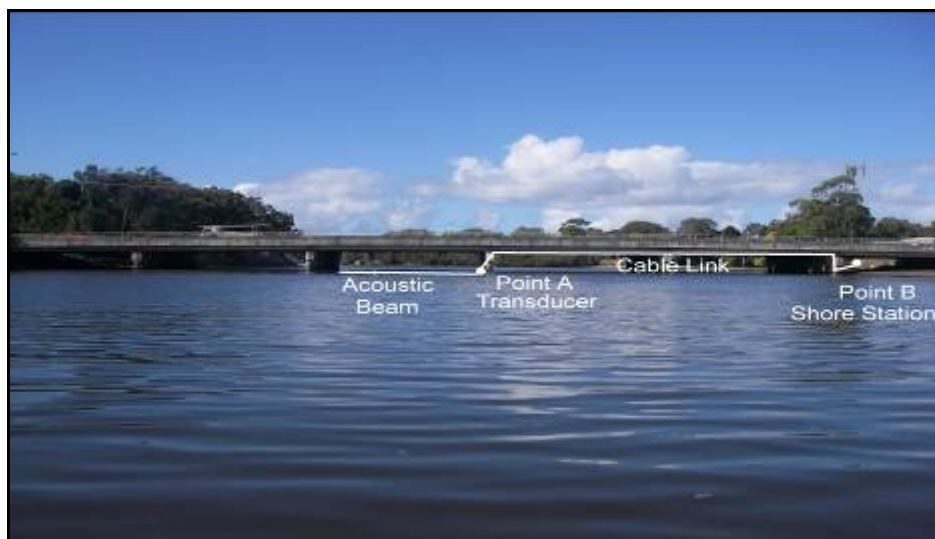
Figure 2. Side View of Currimundi Bridge
