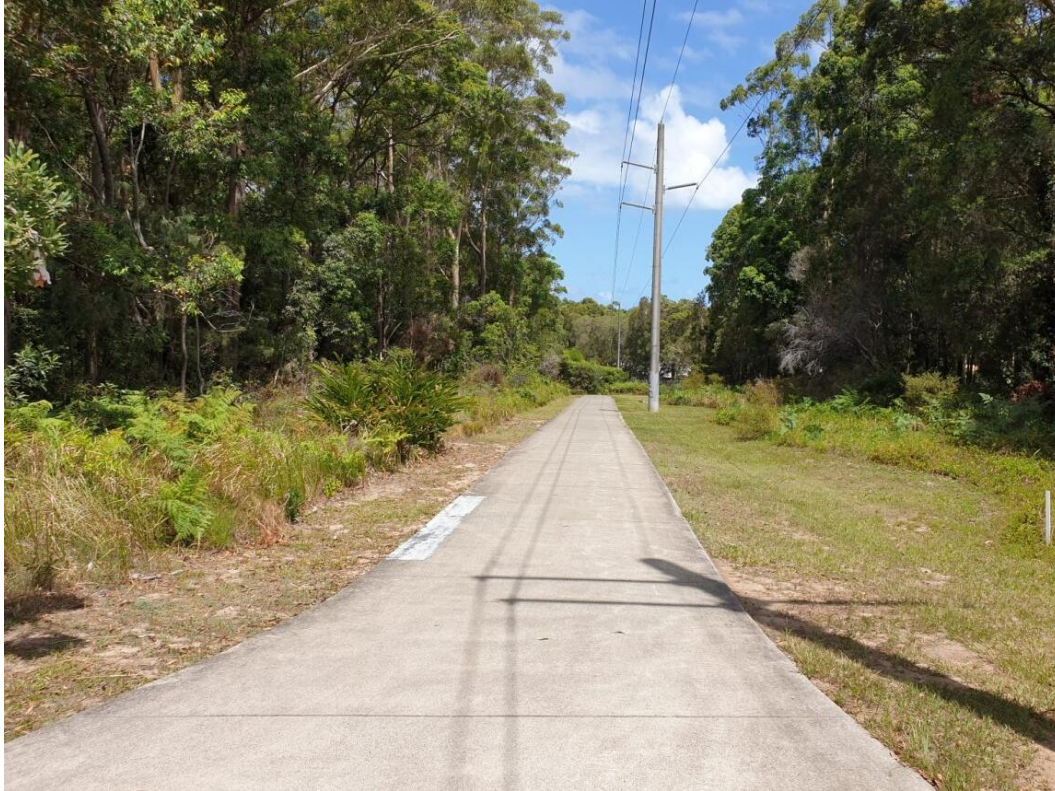
Photograph 2.2 Electricity easement and existing pedestrian path within the Project disturbance footprint (from Nicklin Way looking towards Third Avenue)
