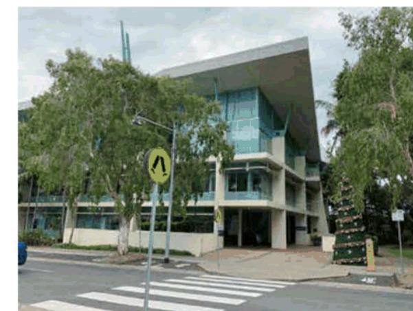
Caloundra Administration Building 2019
