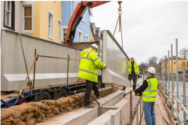
Figure 29 Large scale passive flood barrier system – panel installation A ([www.globalfloodds.com](http://www.globalfloodds.com))
