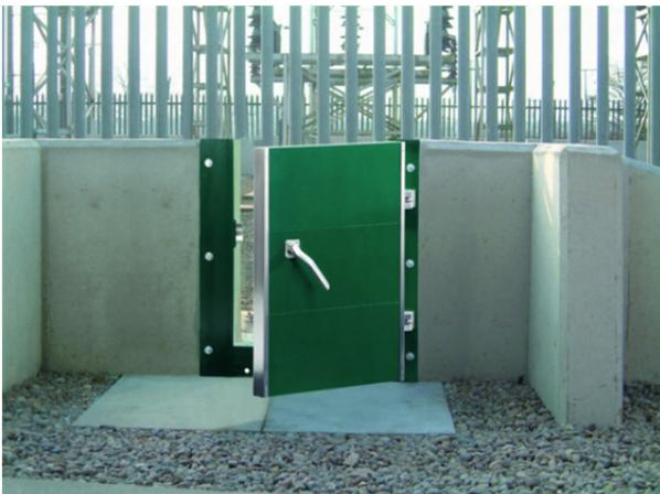
Figure 39 Utility application of a flood door
