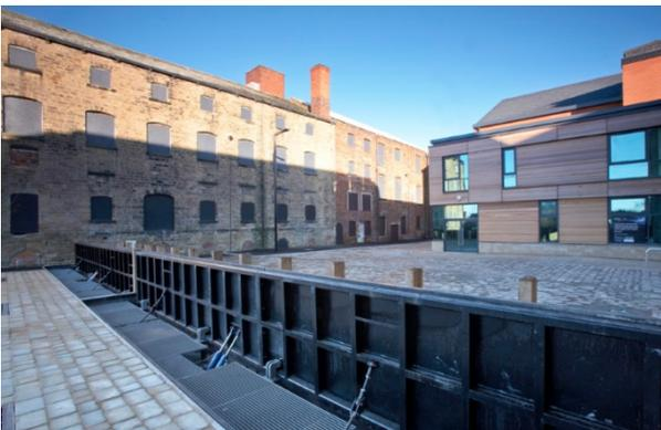
Figure 26 Flip-Up activated flood barrier example ([www.aquobex.com/products/flip-upbarrier](http://www.aquobex.com/products/flip-upbarrier))
