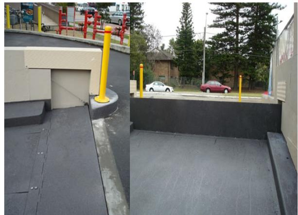
Figure 28 Flip-Up activated flood barrier for basement carpark entrance example ([www.floodingsolutions.com.au](http://www.floodingsolutions.com.au))
