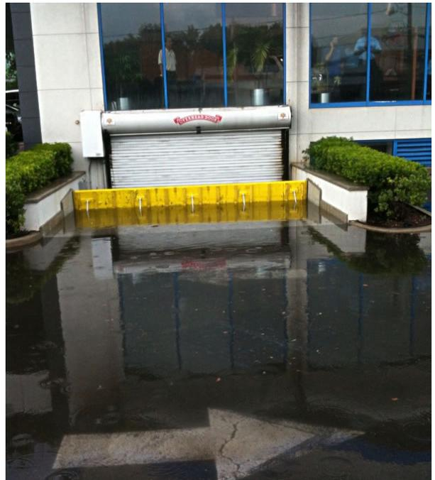
Figure 33 Passive flood barrier system – basement carpark entrance ([www.flood-barriers.com](http://www.flood-barriers.com))
