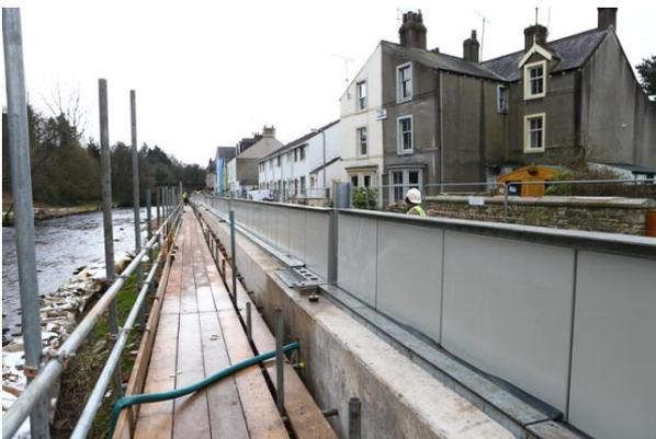
Figure 30 Large scale passive flood barrier system – panel installation B ([www.globalfloodds.com](http://www.globalfloodds.com))
