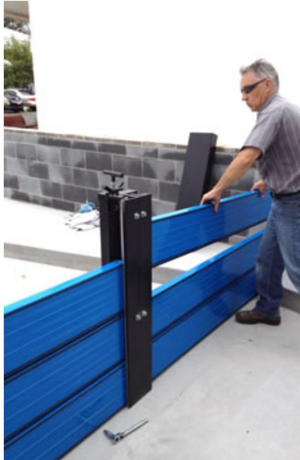
Figure 48 Temporary demountable flood gate
