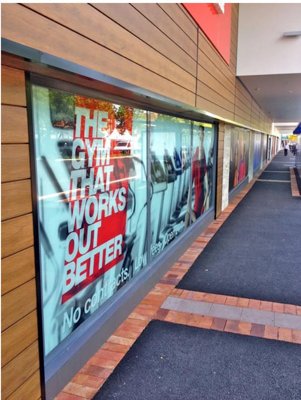
Figure 51 Flood resistant glazing ([www.floodingsolutions.com.au/flood-windows](http://www.floodingsolutions.com.au/flood-windows))
