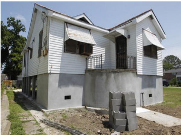
Figure 14 Raised timber framed house with flood resilient lower level building materials
