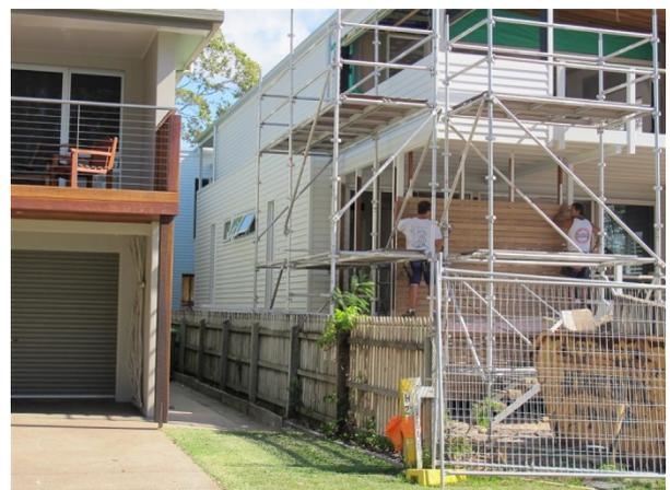
Figure 16 Highset house construction with raised lower floor level
