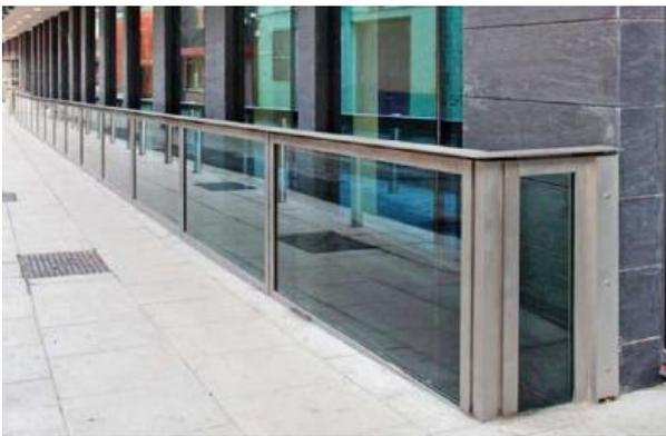
Figure 50 Glass flood protection panels – commercial application ([www.floodcontrolinternational.com](http://www.floodcontrolinternational.com))
