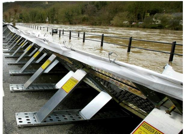
Figure 25 Temporary rigid flood barrier ([www.hydroresponse.com](http://www.hydroresponse.com))
