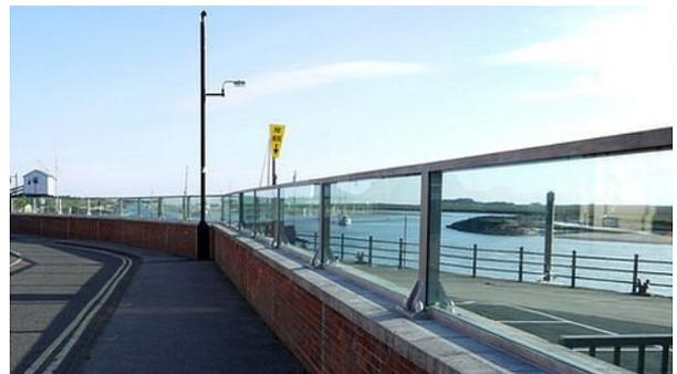
Figure 36 Permanent glass flood protection panels – public flood defence system application ([www.floodcontrolinternational.com](http://www.floodcontrolinternational.com))
