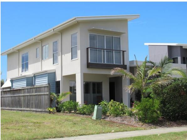
Figure 17 Slab on ground lower level with second storey flood retreat area
