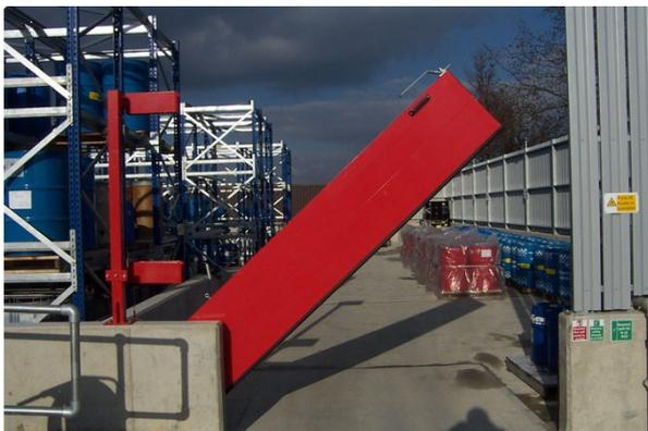
Figure 45 Side vertical pivoting flood gate
