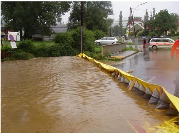
Figure 24 Temporary flexible flood barrier ([www.hydroresponse.com](http://www.hydroresponse.com))
