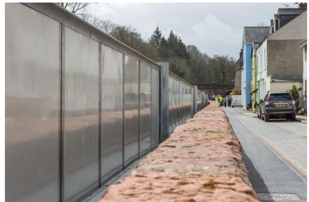
Figure 32 Large scale passive flood barrier system – panel engaged ([www.globalfloodds.com](http://www.globalfloodds.com))
