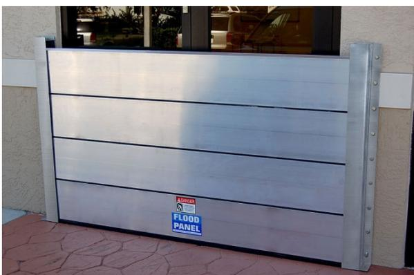
Figure 47 Temporary demountable flood gate
