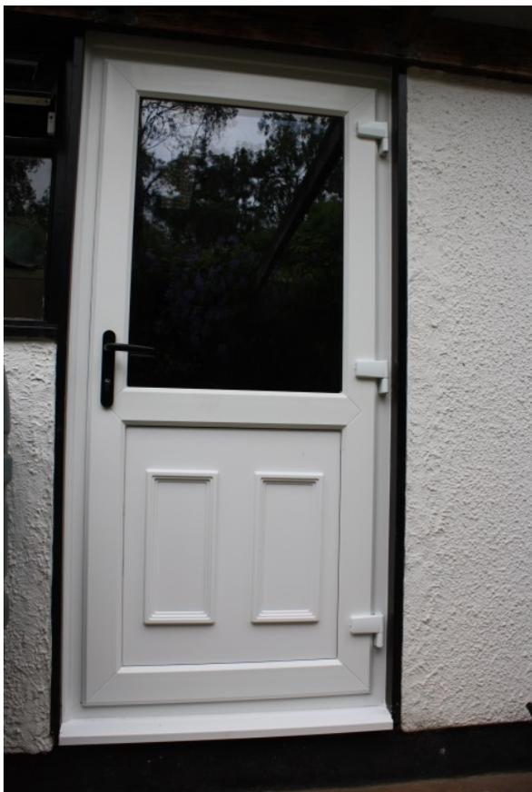
Figure 41 Domestic flood door application ([www.doorfactory.co.uk](http://www.doorfactory.co.uk))
