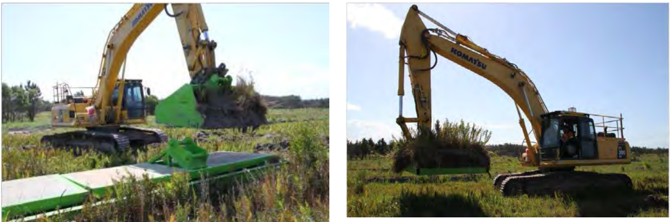
Photograph 2: Example heath tile translocation methodology employed by Shadforths Civil Contractors.
