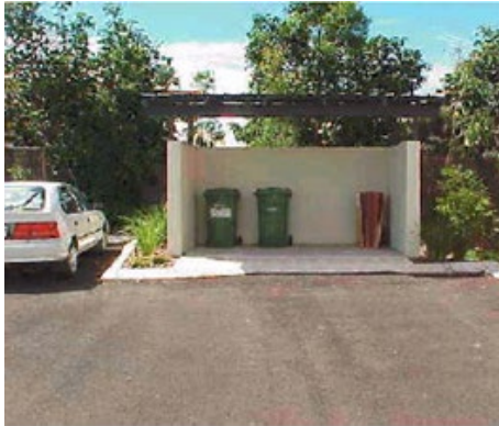
Roofed waste storage container area for 240 litre bin type.
