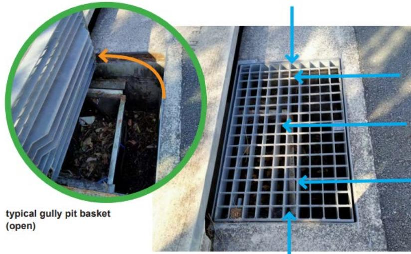
Spatial Relationship: A GPT Simple asset’s spatial location must correlate with a Pit/Manhole asset as they are housed within those structures and can be removed for maintenance or relocation.
