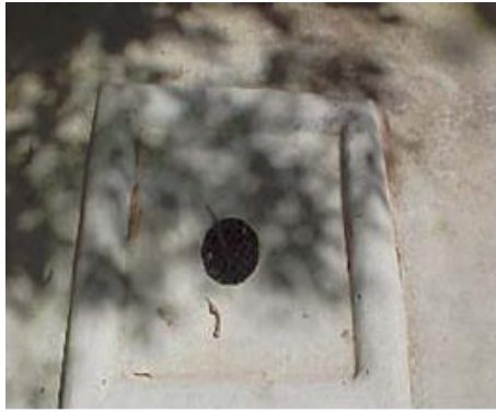
Bunded bin wash down area in further detail.
