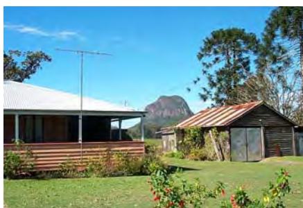
Shed and Garage
