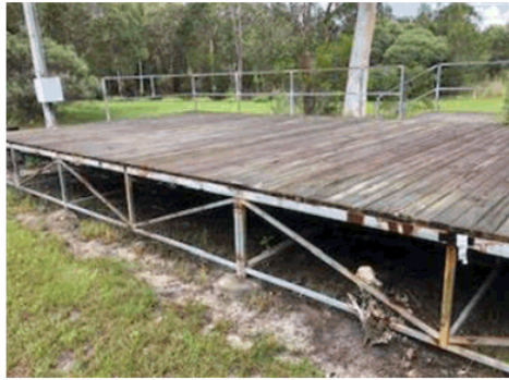
Stage & Retaining Wall
