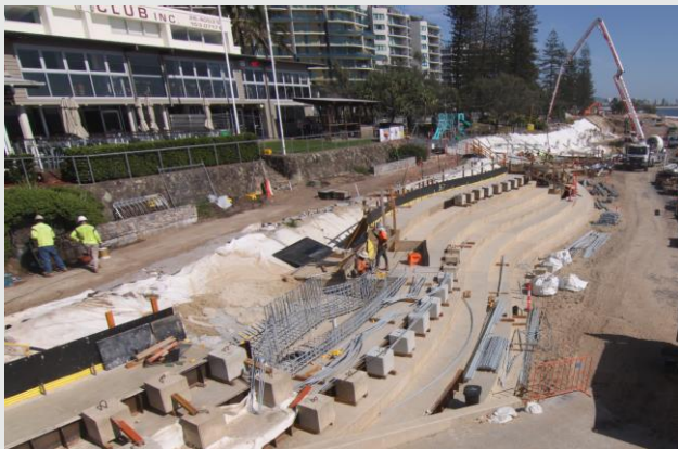
Figure 1 Replacement seawall under construction
