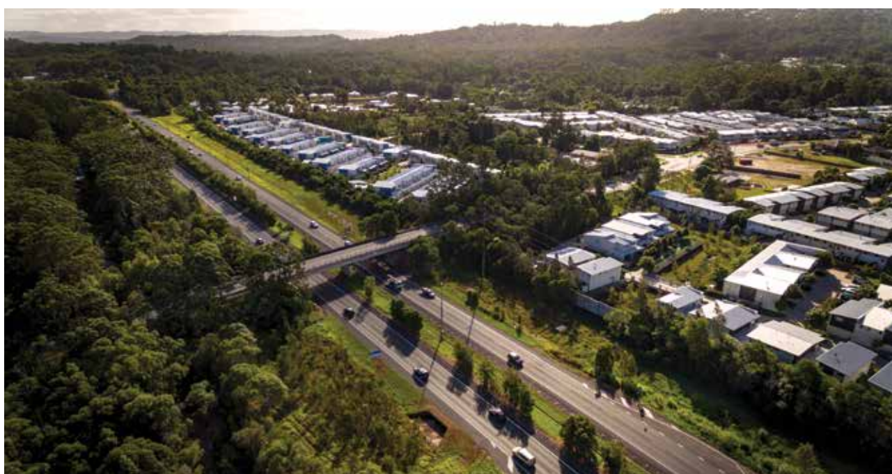
Residential development in Buderim
