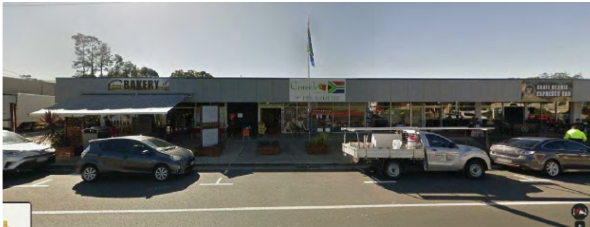
Figure 15 – view of the existing Forest Glen Shops fronting Mons Road
