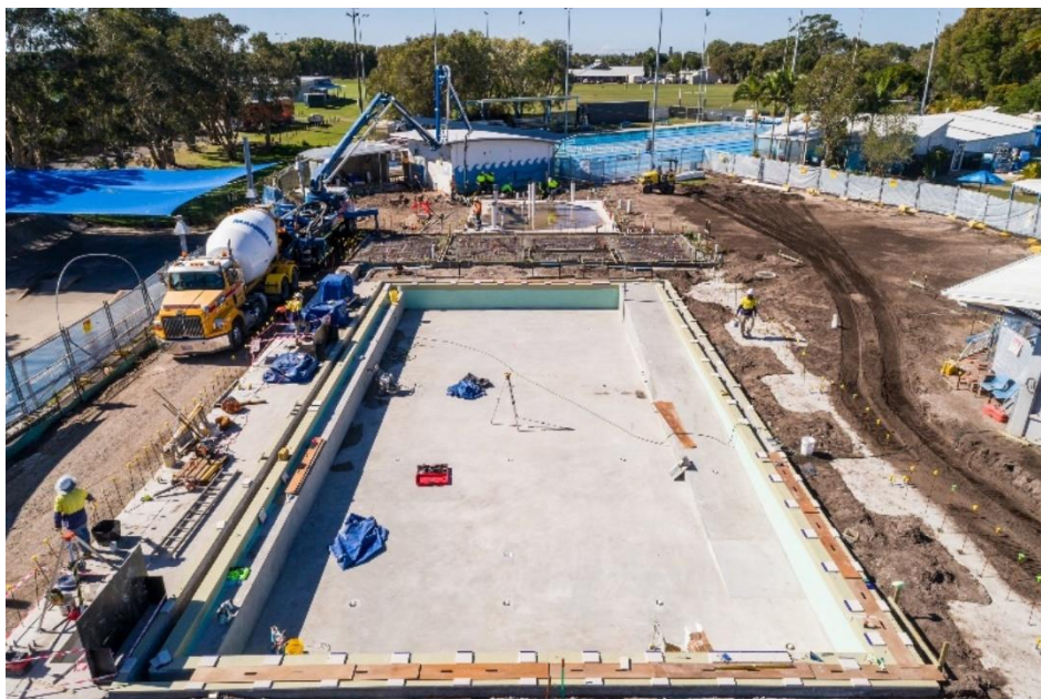
Figure 1: The new indoor program pool under construction
