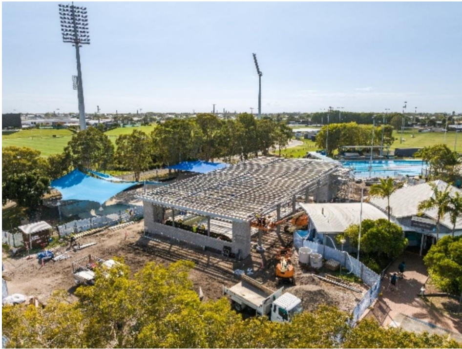
Figure 2: The new indoor program pool structure under construction
