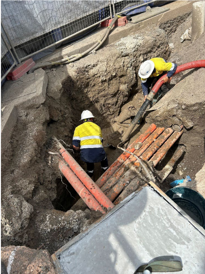
Figure 2. New water main excavation works.
