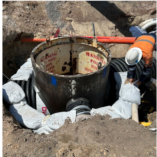
Figure 2. Major stormwater and drainage works installing stormwater pipes of 900mm diameter.
