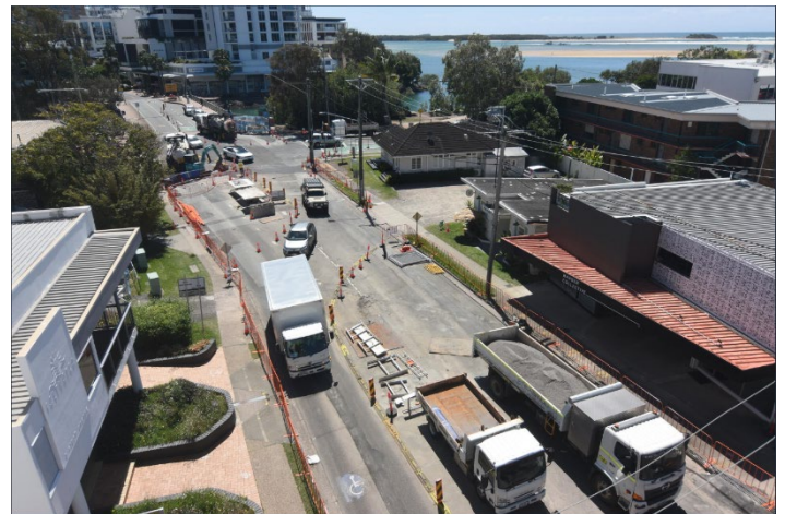
Figure 1. First Avenue works zone with pedestrian and southbound traffic and access to businesses remaining.
