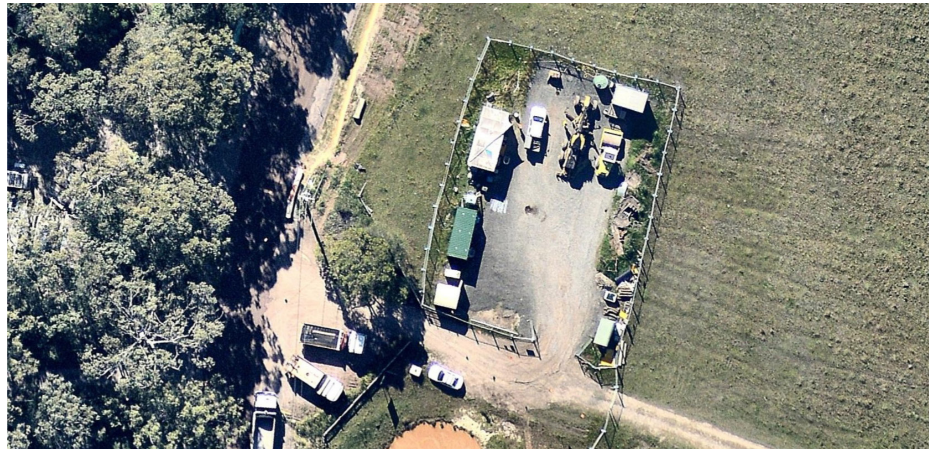
Existing site storage area at Doonan Bridge Road.
